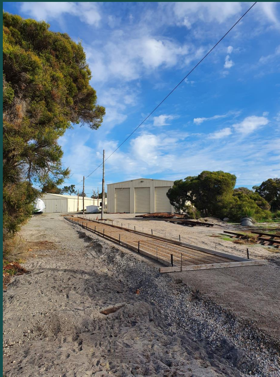
Formwork for the raft.
