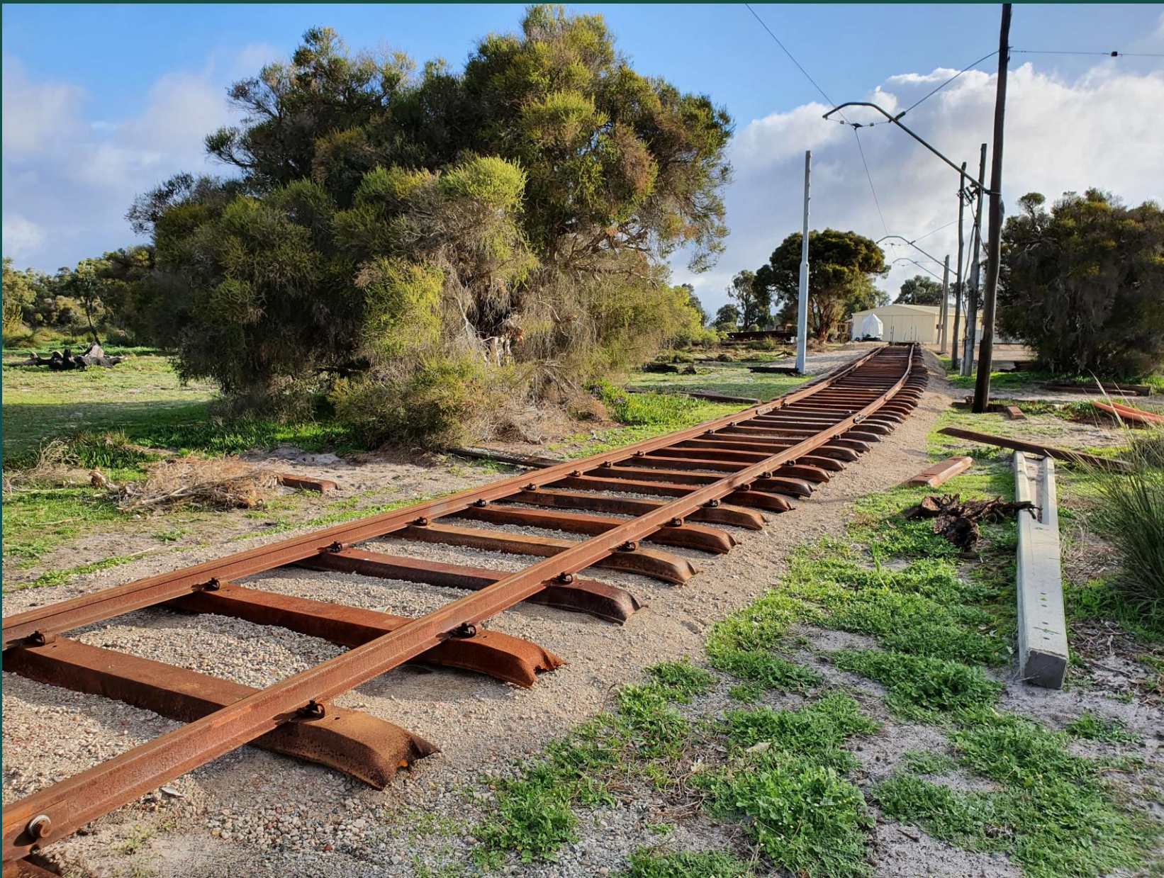
Steel sleepers and rail in place on the ramp.
