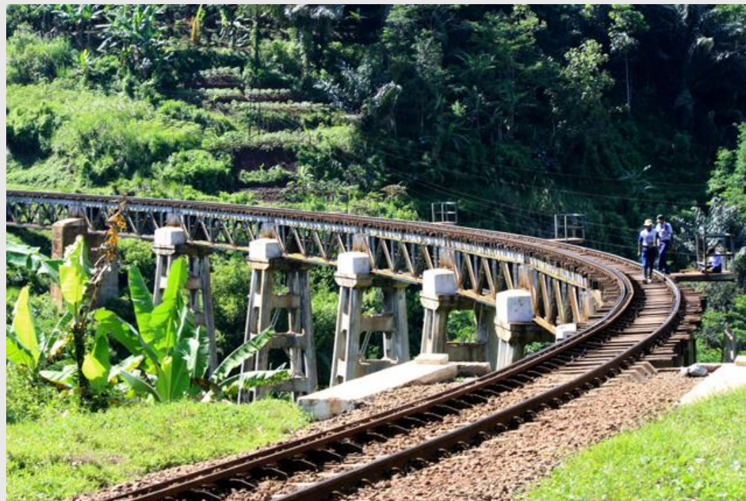
Ciharang Bridge between Bumiwaluya and Cipendeuy Stations.
