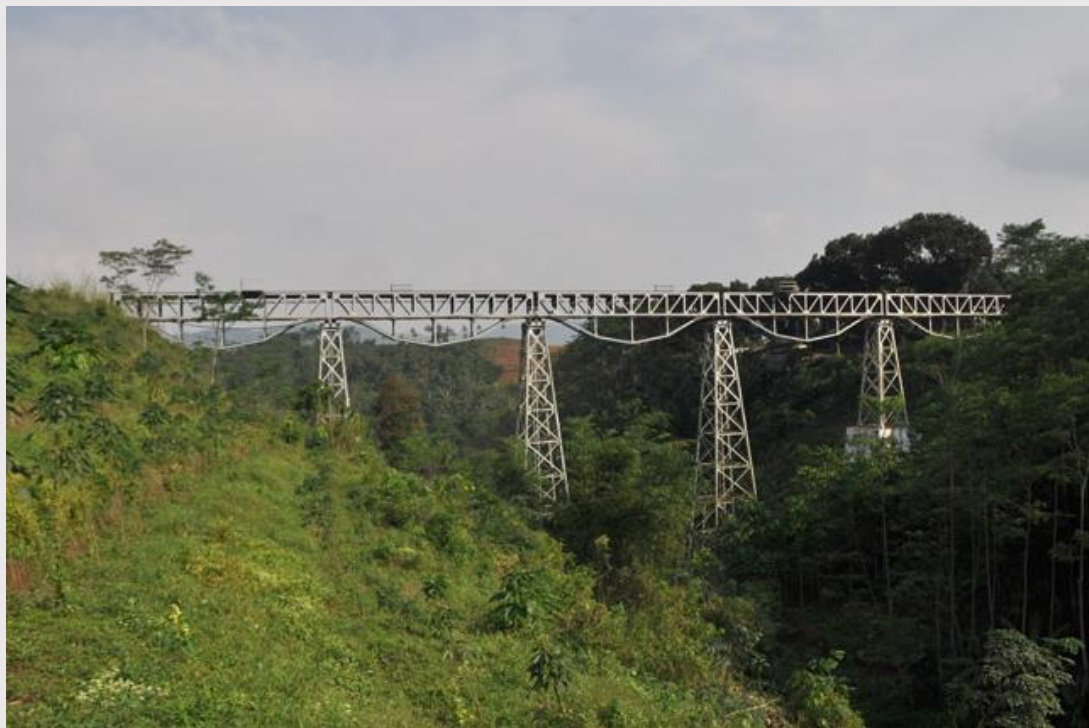
Cirangrang Bridge between Sasaksaat and Cilame Stations.
