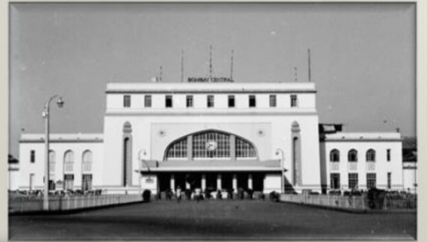
MUMBAI CENTRAL 1930 Architect: Claude Batley
