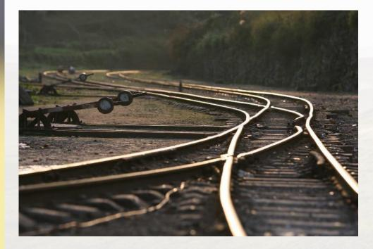
The narrow-gauge (762mm) railway line on which the little train runs is between Bajiaogou town and Shixi town in Qianwei County, which is 12 km from the county seat of Qianwei. Total length of the track is 19.84km and there are 6 tunnels and 108 curves with minimum radius of 70m, maximum gradient at 36.14‰ and a difference of 238m in elevation along the line.
